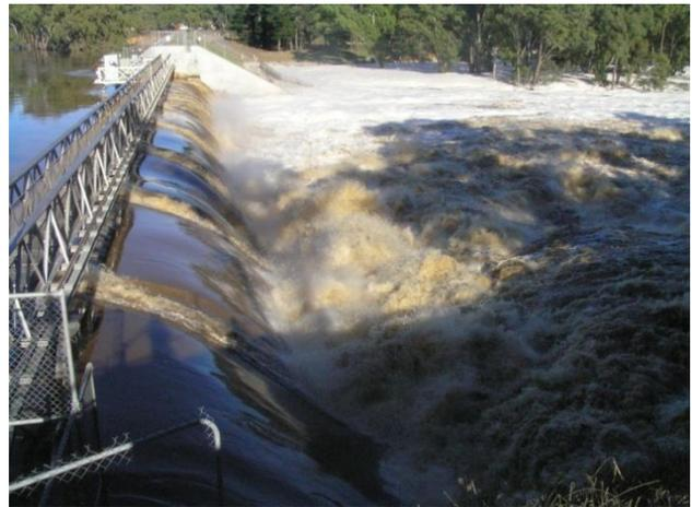
**Figure 6 – Laanecoorie Dam in January 2011 Flood. Remedial works at the embankment /spillway interface carried out in 2009 were tested during the second rank flood in recorded history on the Loddon River**
