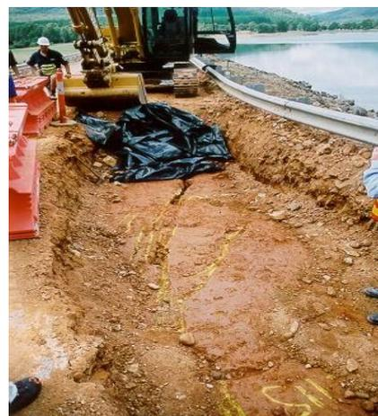
**Figure 1 – Cracking discovered in Buffalo Dam core during site investigations (2001)**
